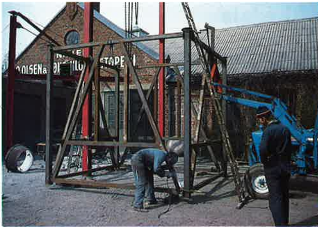
Custom steel fabrication.
